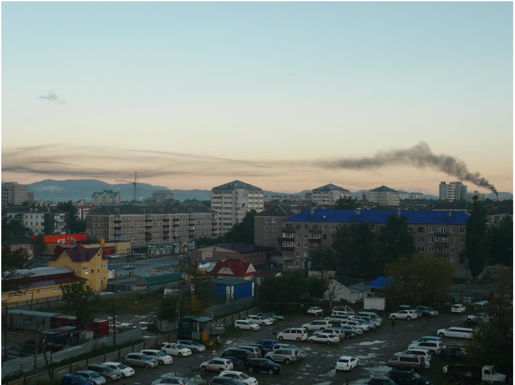
Smoke from Heat Power plant chimney in Yushno-Sakhalinsk on September 19, 2011
